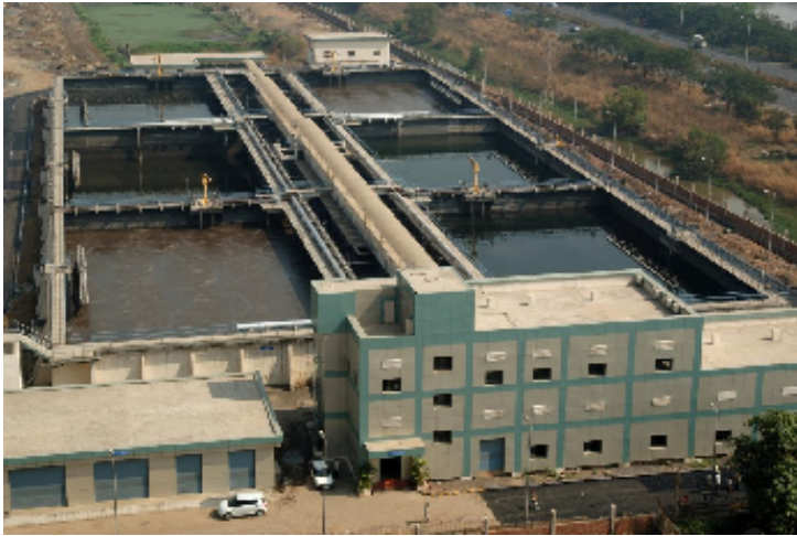
Figure 2: NERUL STP 3 X 2 BASIN MODULES, 100 MLD design
