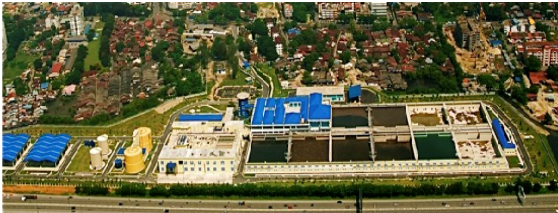
Figure 3: JELUTONG STP 3 x 4 BASIN MODULES; 22,500 kg BOD/d and 90,000 m 3 /d EACH MODULE DESIGN
