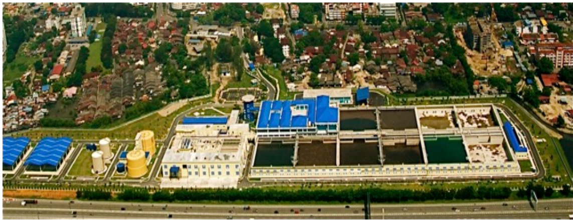
Figure 1: C-Tech configured sequencing batch reactor – Jelutong STP
